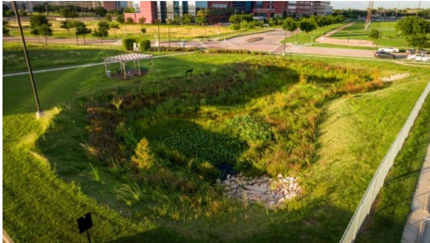
Parking lot transformed into a stormwater retention pond at MD Anderson Cancer Center in Houston, Texas
