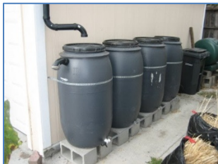
200 gallons of storage tucked next to a garage
